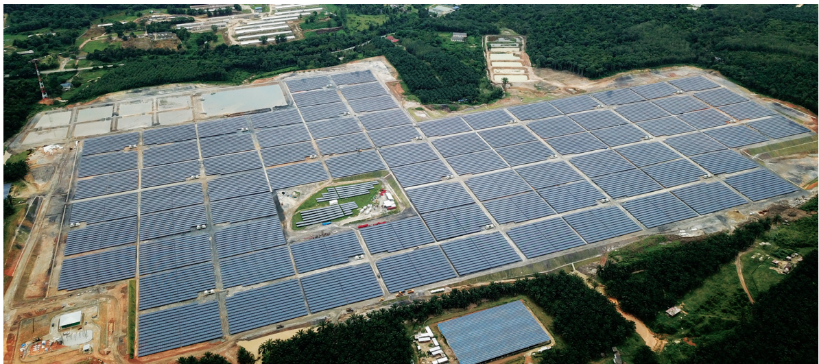
Solar farm at Rembau, Negeri Sembilan
