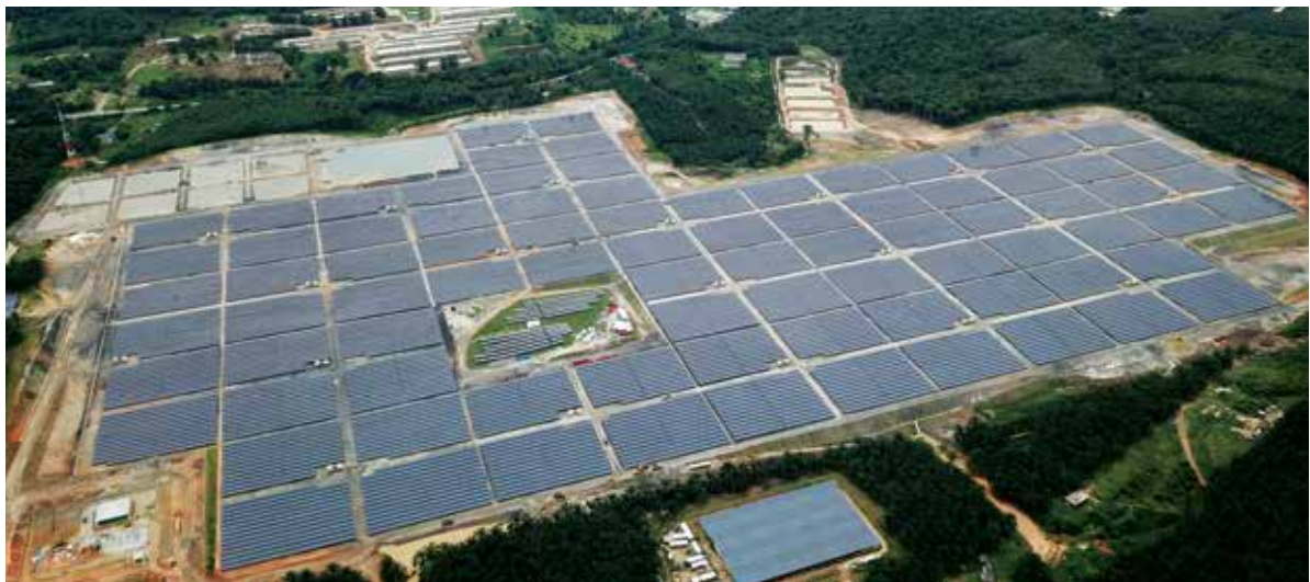
Solar farm at Rembau, Negeri Sembilan
